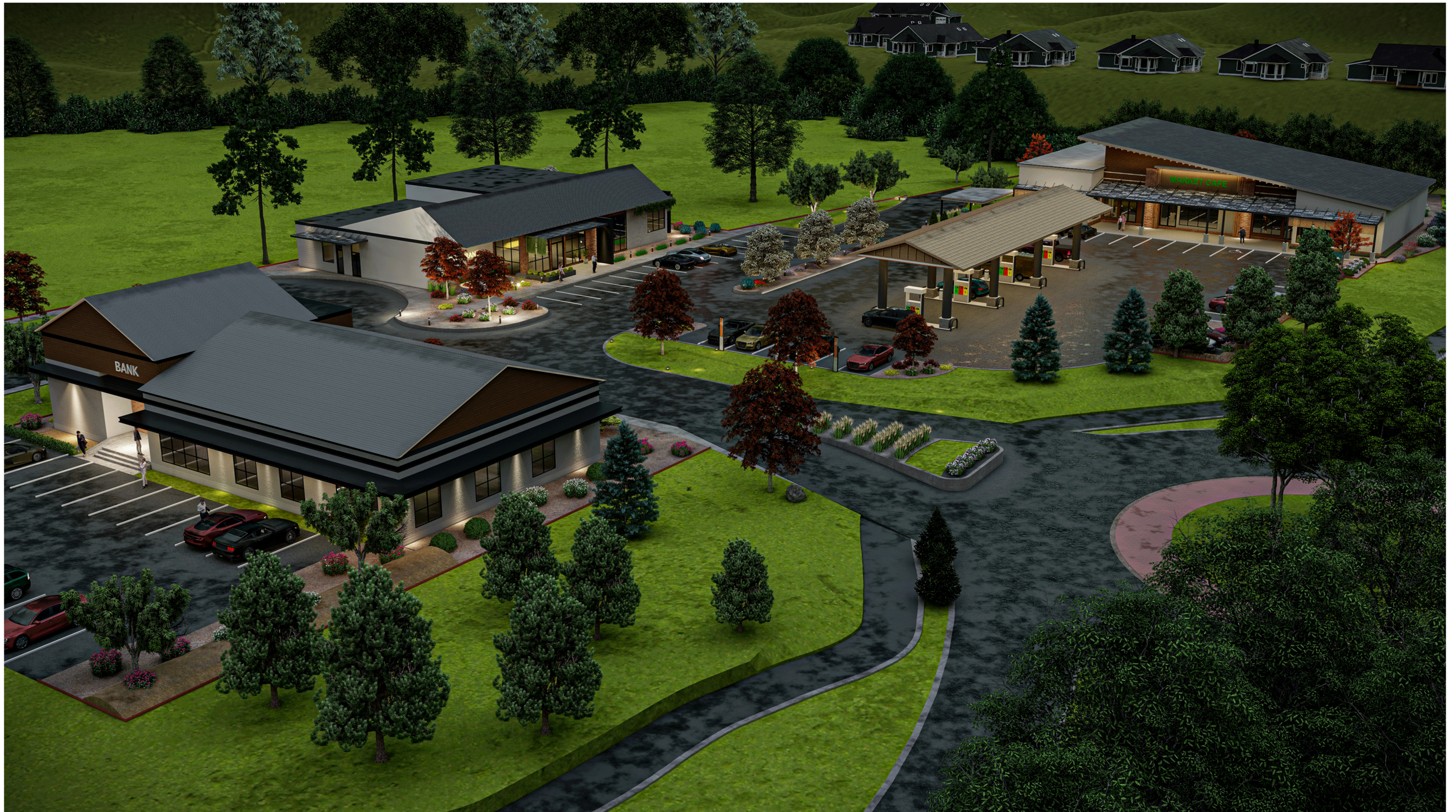
Site Aerial View - Night
