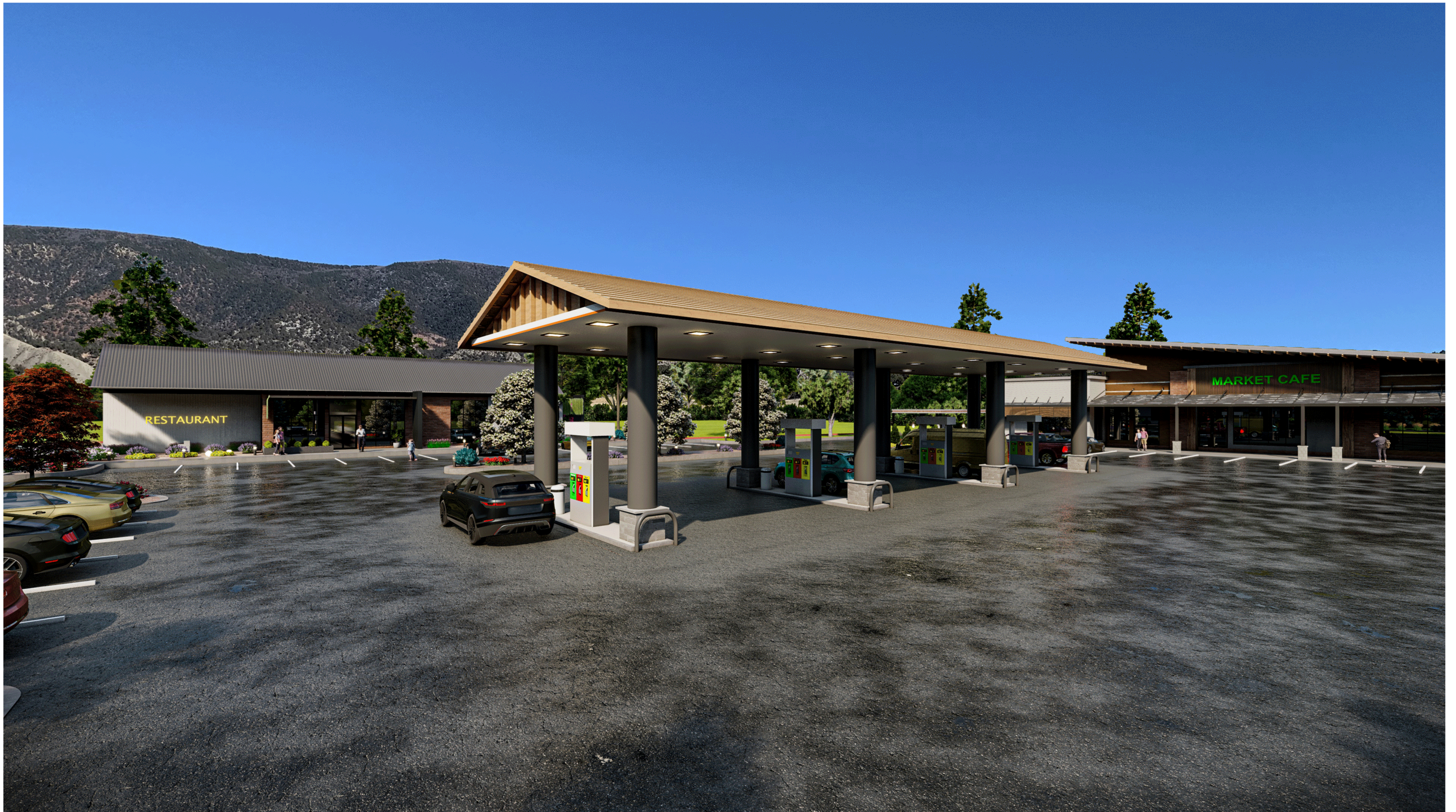
View F - Fuelling Shed/Gas Station
