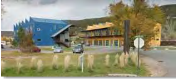
Mid-Valley Design Center Live-Work
